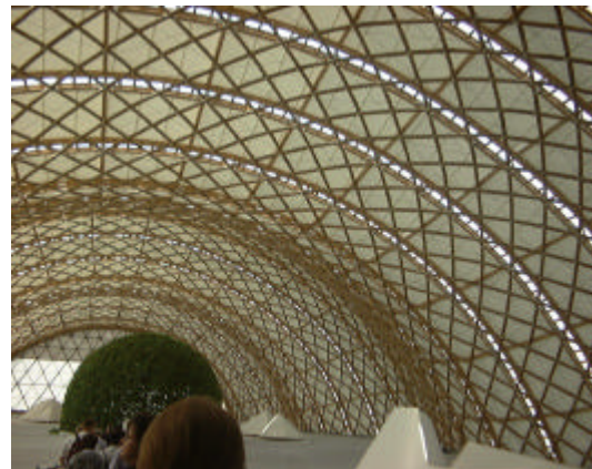
Japan pavilion made entirely of several-hundred-foot long cardboard tubes and resin-coated paper
