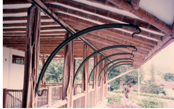
Art nouveau detailing with rebar
