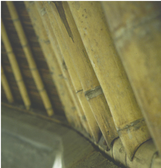
“Fish-mouth” joints on both ends of a line of poles make precision a necessity.
