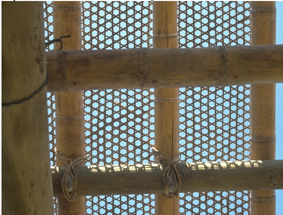
This view is up at a ceiling through the palm mat lath.
