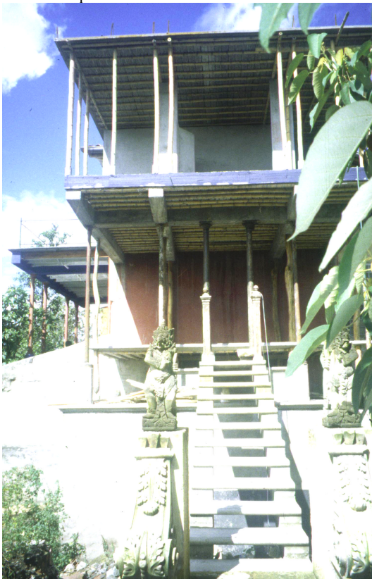
Velez' new office under construction
